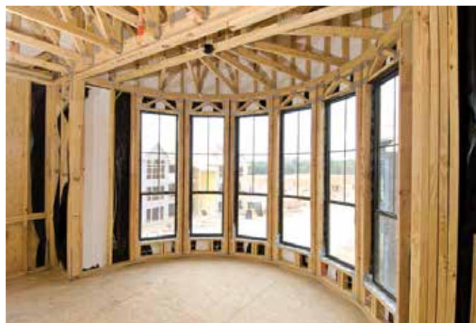
Harris says like traditional wall, roof and floor components, its plated headers, corners and other rough openings offer builders and framers tremendous value in many areas.
